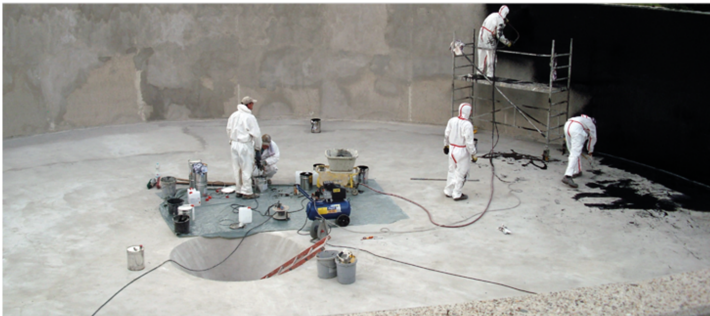
BASIN RENOVATION Treatment plant, Calbe
