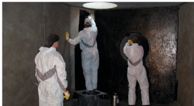
MAIN CHAMBER RENOVATION Rainwater retention basin, Birkenwerder
